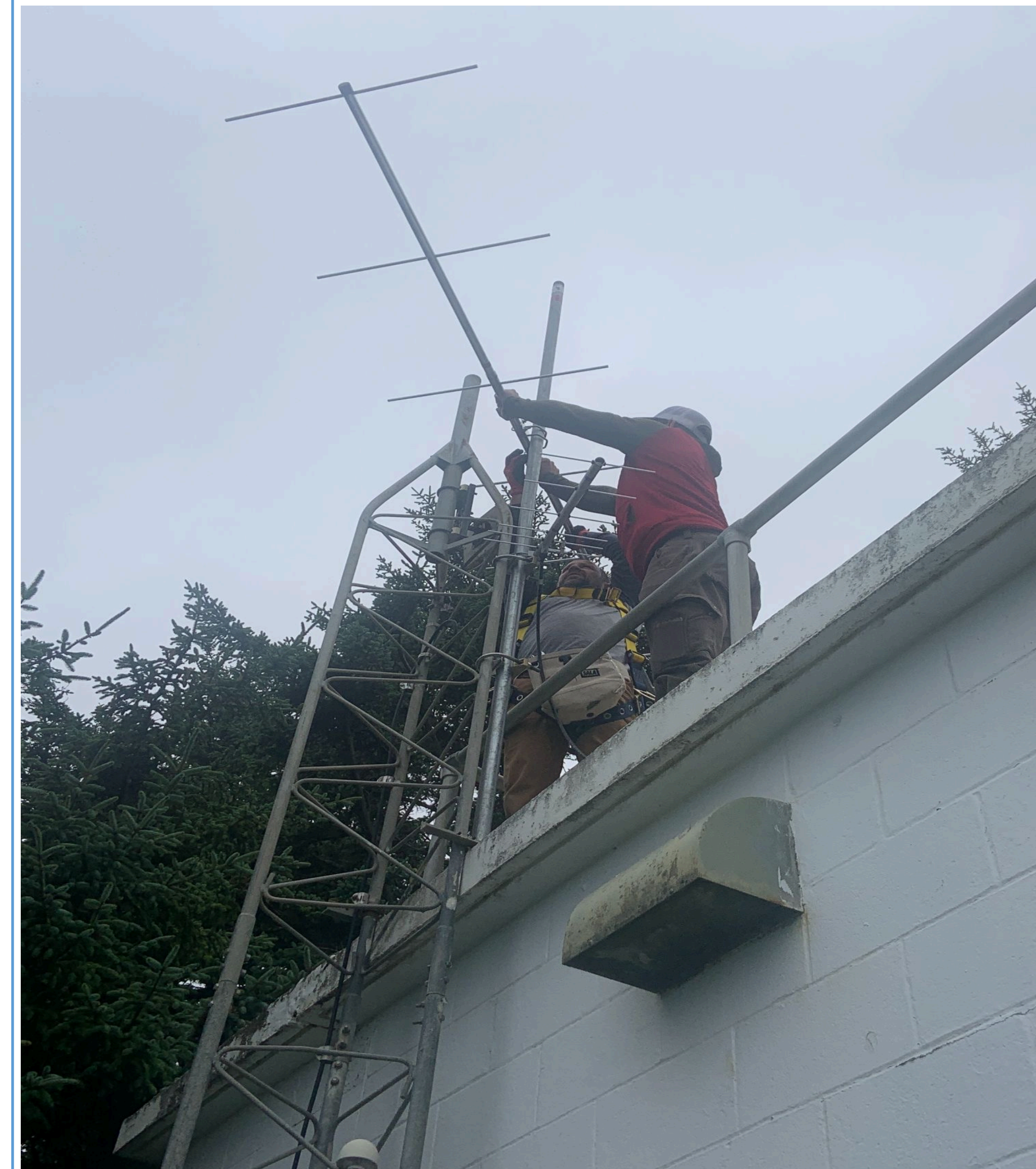
Image 4: Installation of the Cape Meares Antennas
