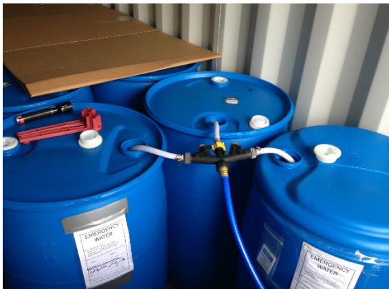
Figure 44: Filling Three 55-gallon Water Barrels
