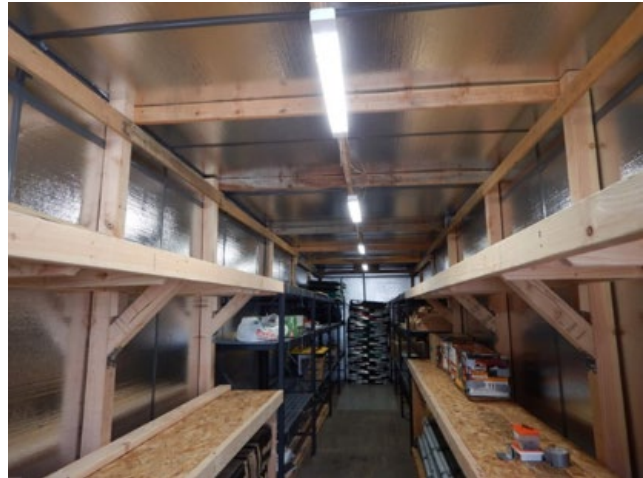
Figure 17: Reflective Foil Core Insulation Photo courtesy of Jim Buck
