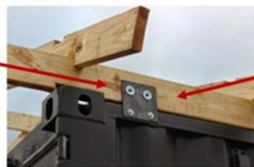
Weld 10 each 6"x6" x 1/4" thick steel plates at locations shown on sketch.
